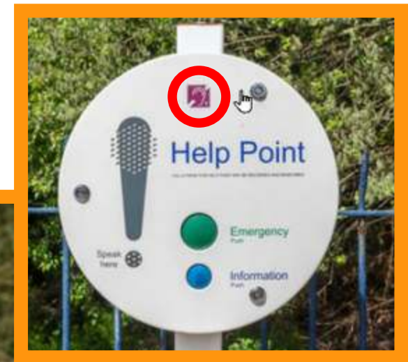
Looped emergency help point in parking
